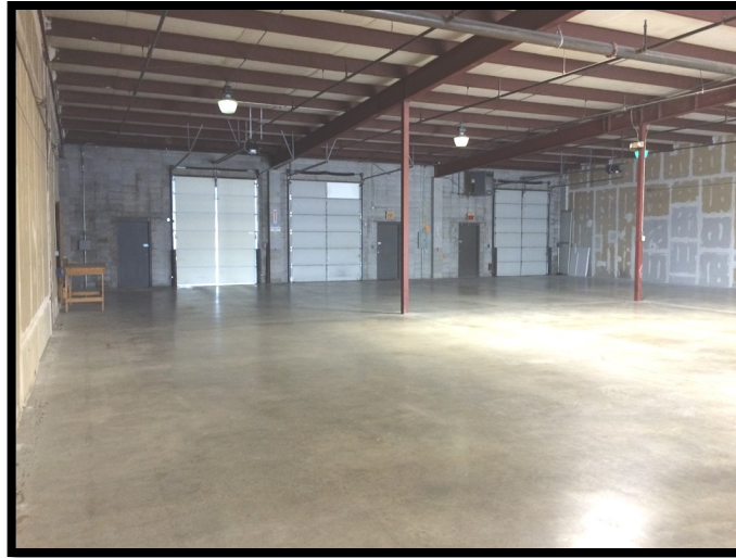
3045 C-D Warehouse (North View)
